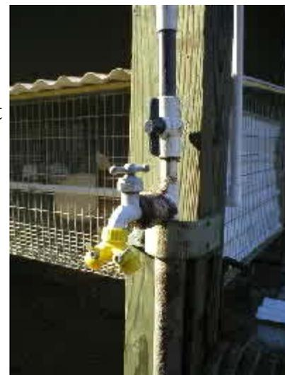
Hang your pipe first - DO NOT drill holes first. I've found there is nothing gained by drilling first - only frustration when things don't line up right later. Place your pipe at least 8 inches high in the cage. Sounds high but it's not. Secure your pipe to the cages. I used some wire clips from Klubertanz designed to hold electric fencing to fence insulators. A box of 200 or so of these was about \$2.00 and saved me a lot of time and the hassles of cutting, bending, and twisting wire.
